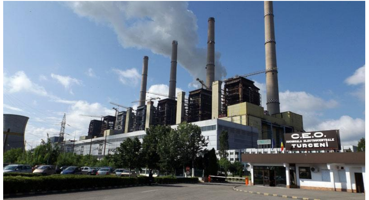
Lignite energy power plant TURCENI
