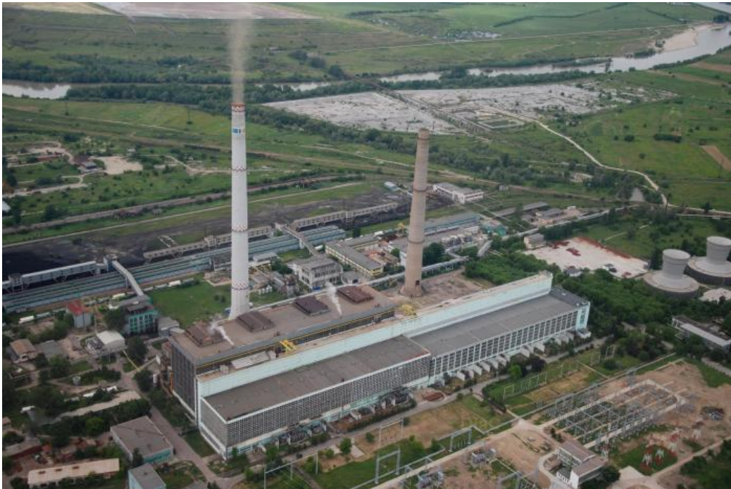
Lignite energy power plant ISALNITA
